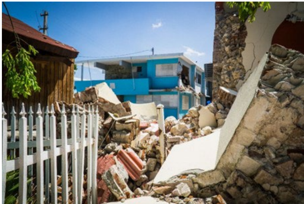
Figure 2: Damage from 6.4 earthquake on January 7, 2020, in Guayanilla
